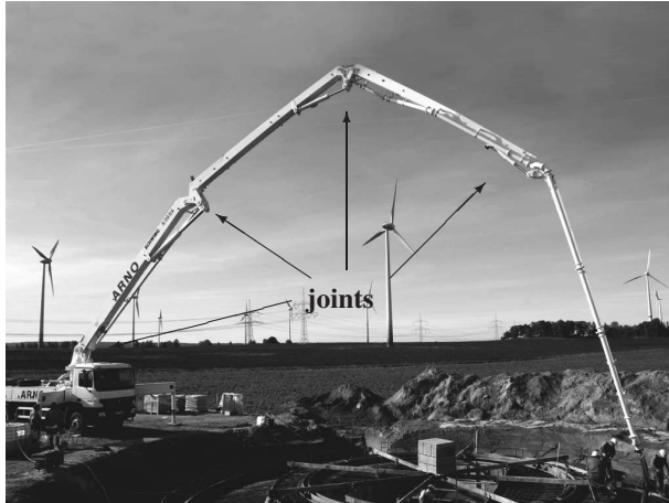
Fig. 1. Mobile concrete pump with four joints.
