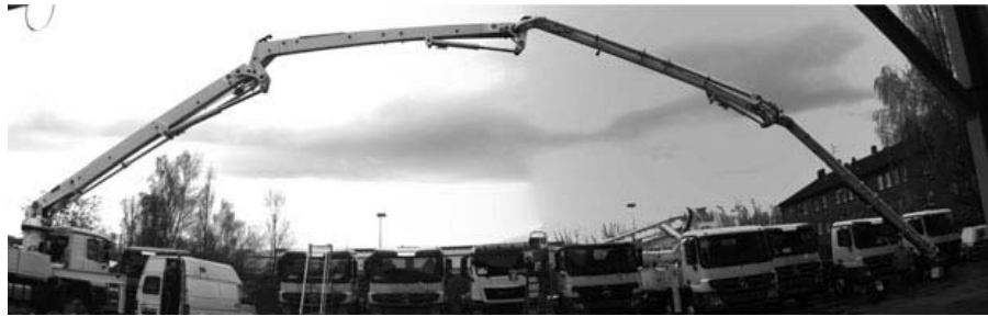
Figure 1. Boom of a mobile concrete pump.
